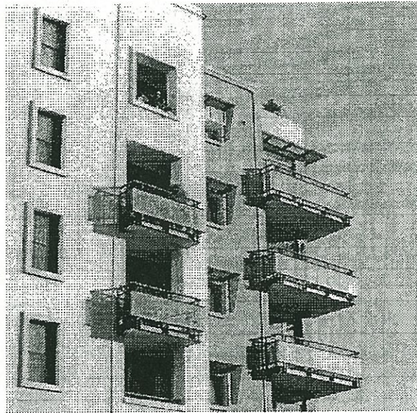
Balconies provide surface articulation and reduce the mass of a facade
