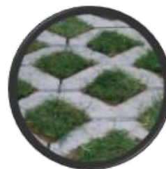
Figure 4 – Example of permeable paving
