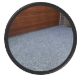
Figure 5 – Example of permeable concrete/ asphalt
