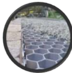
Figure 3 – Example of plastic grid system
