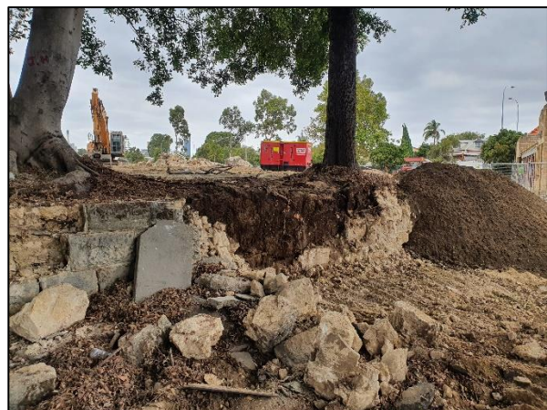
Image 6 – Limestone wall removal
