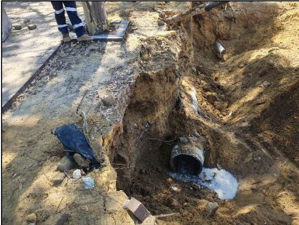
Image 5 – Storm water pipe removal
