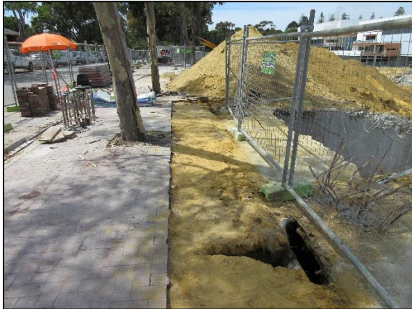
Image 1 – Exploratory vacuum excavation
