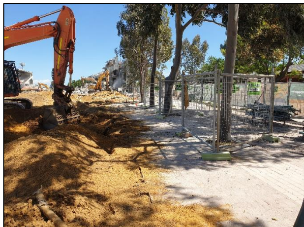
Image 4 – Soil replaced after footing removal
