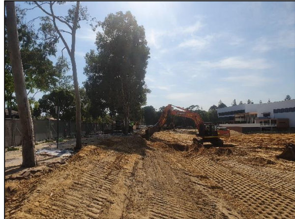
Image 6 – Battering of fill soil post excavation
