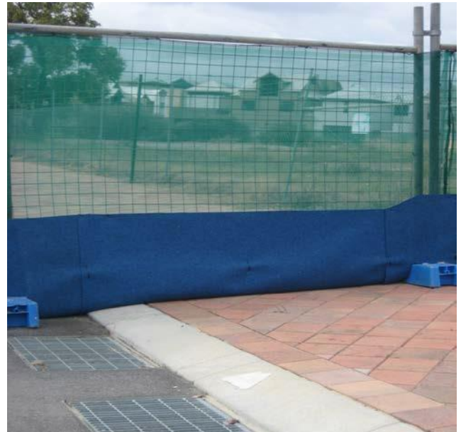
Figure 2: Front view showing sediment control fence protecting stormwater drains.
