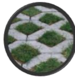
Figure 5 – Example of permeable paving
