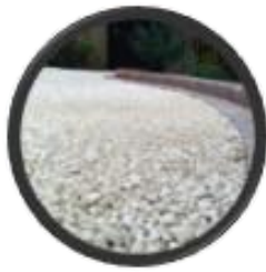
Figure 3 – Loose stone/ gravel driveway
