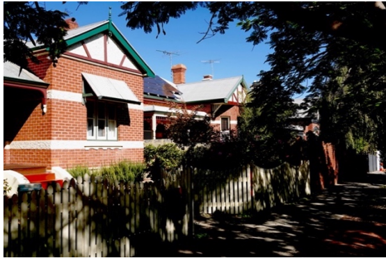
The streetscapes are unified by compatible materials, architectural forms and some key design elements, largely derived from the Federation Queen Anne style.
