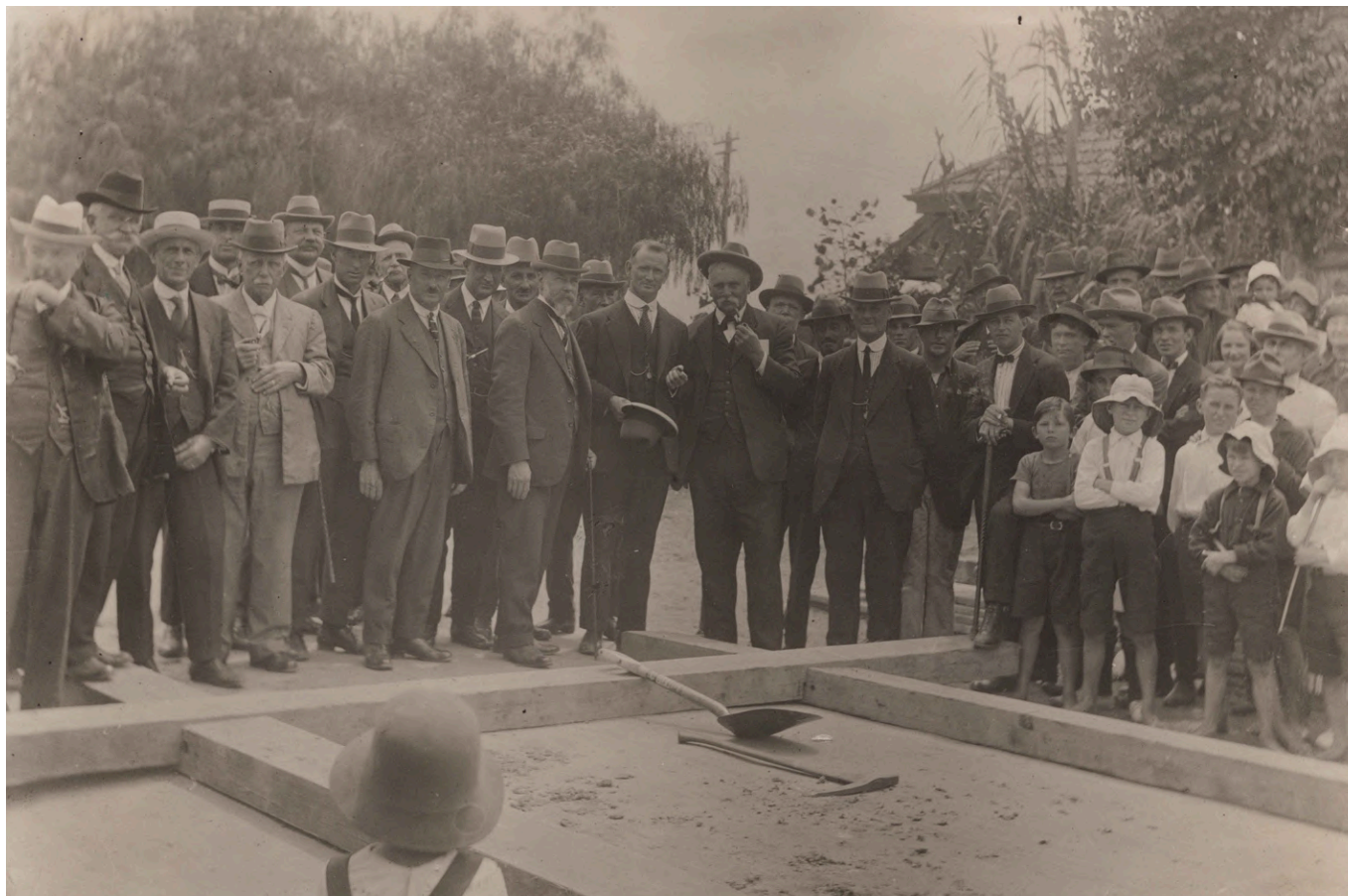
Mayor of Subiaco Roland A. Robinson and officials at the ceremony of the turning of the sod for the installation of the Subiaco sewerage system, circa 1924. (Subiaco Museum Collection).
