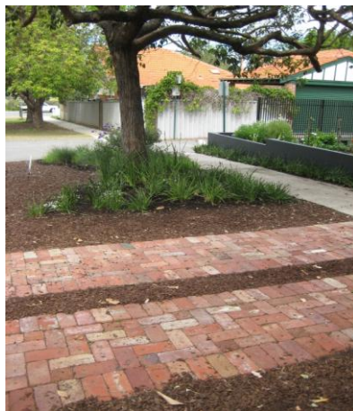
Image: displaying a suitable example of verge paving.
